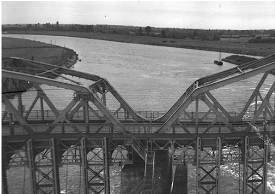
GRAVE ROAD BRIDGE
