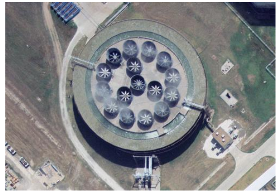
COOLING VENTS, HOUSTON
