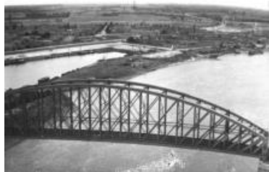
NIJMEGEN RAIL BRIDGE
